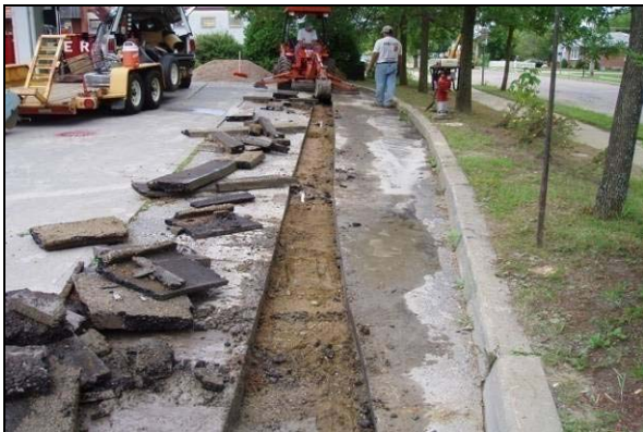
Figure 1. Trenching for installation of the subsurface conveyance piping.
