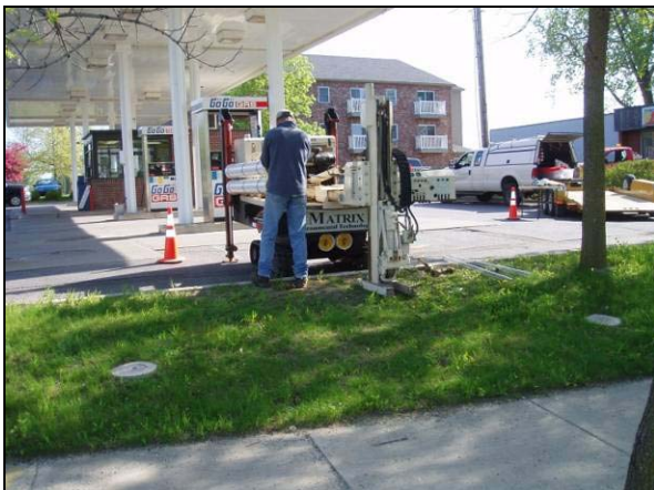
Figure 2. Installation of oxygen injection points using a Geoprobe®
