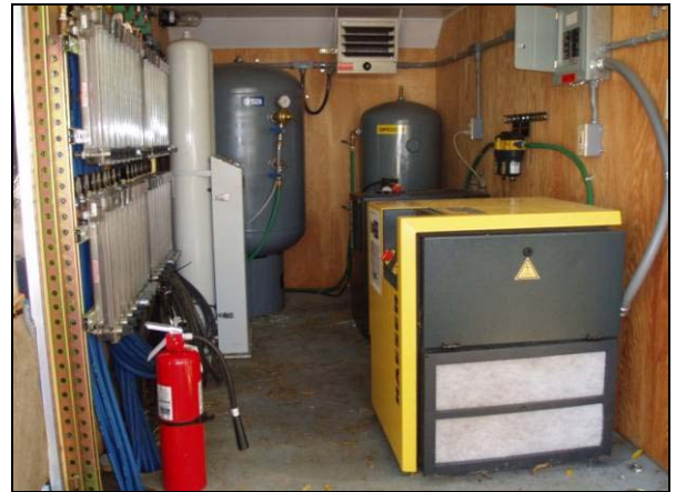
Figure 3. Oxygen Injection System
