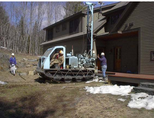
Figure 2. Subsurface Investigation using Track-Rig
