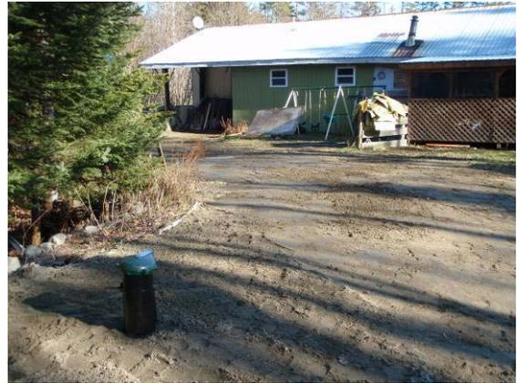
Figure 3. New bedrock supply well installed to replace impacted spring
