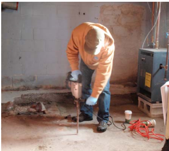
Figure 1. Installing vapor sampling point beneath a concrete floor
